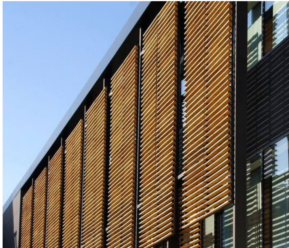
Wood and steel facade screen
